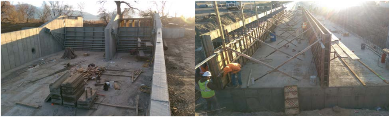
Little Weber Diversion Structure
