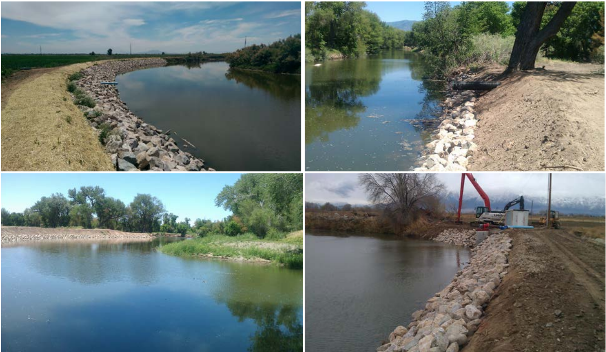
Lower Weber River Bank Stabilization and Repair
