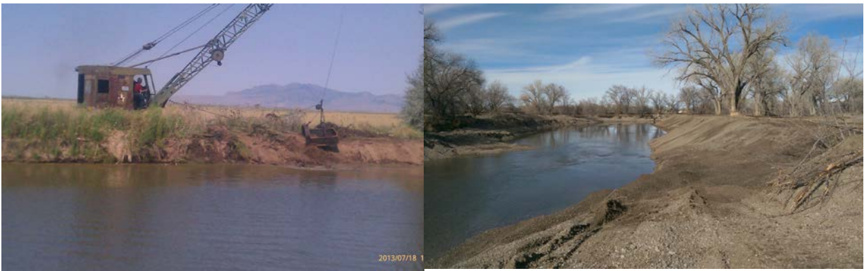
Silt and Debris Removal Efforts
